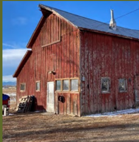
Murray-Culver Farm: barn
