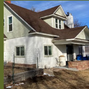
Murray-Culver Farm: house
